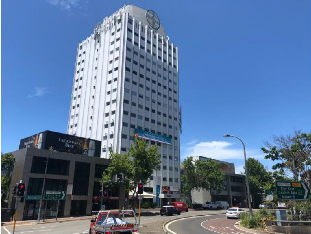
Figure 3: View from the north west 283 Walker Street (left), 275 Walker Street (centre) and 271-273 Walker Street (right) (Source: Mecone)
